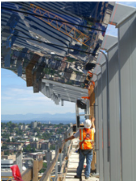
Installing the Blue Glass Canopy
